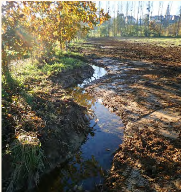
Water way rewinding work
